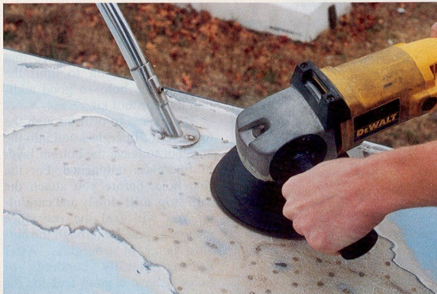
After you've filled the void with epoxy, sand smooth and apply primer, paint and nonskid.
